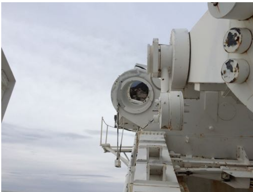
Figure 7.4: Looking up towards McMath's 0.9 m West Auxiliary Heliostat. This is the last optic in the chain before the beam is sent to the observing telescope
